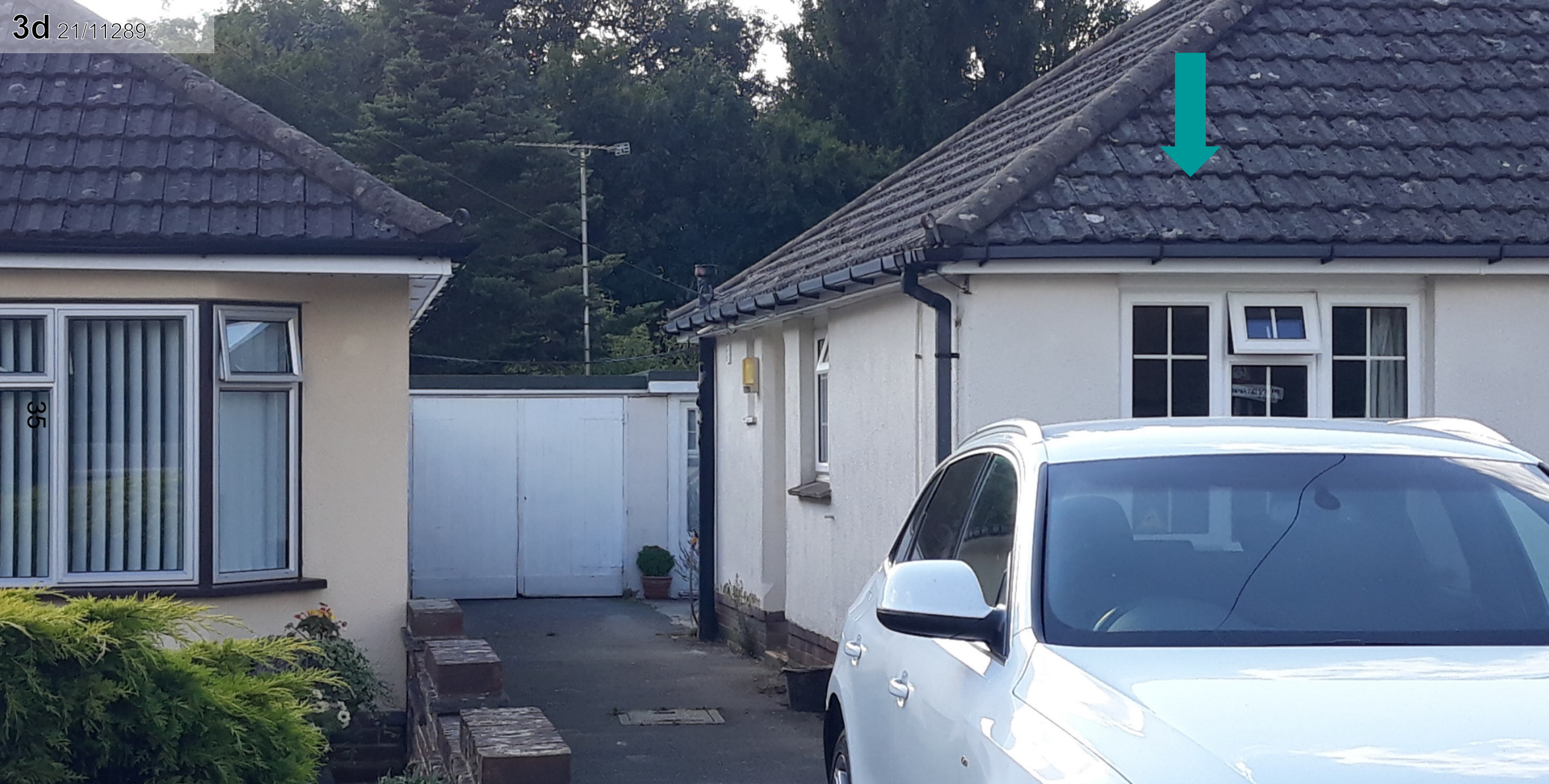
33 Close up of side elevation showing backdrop
