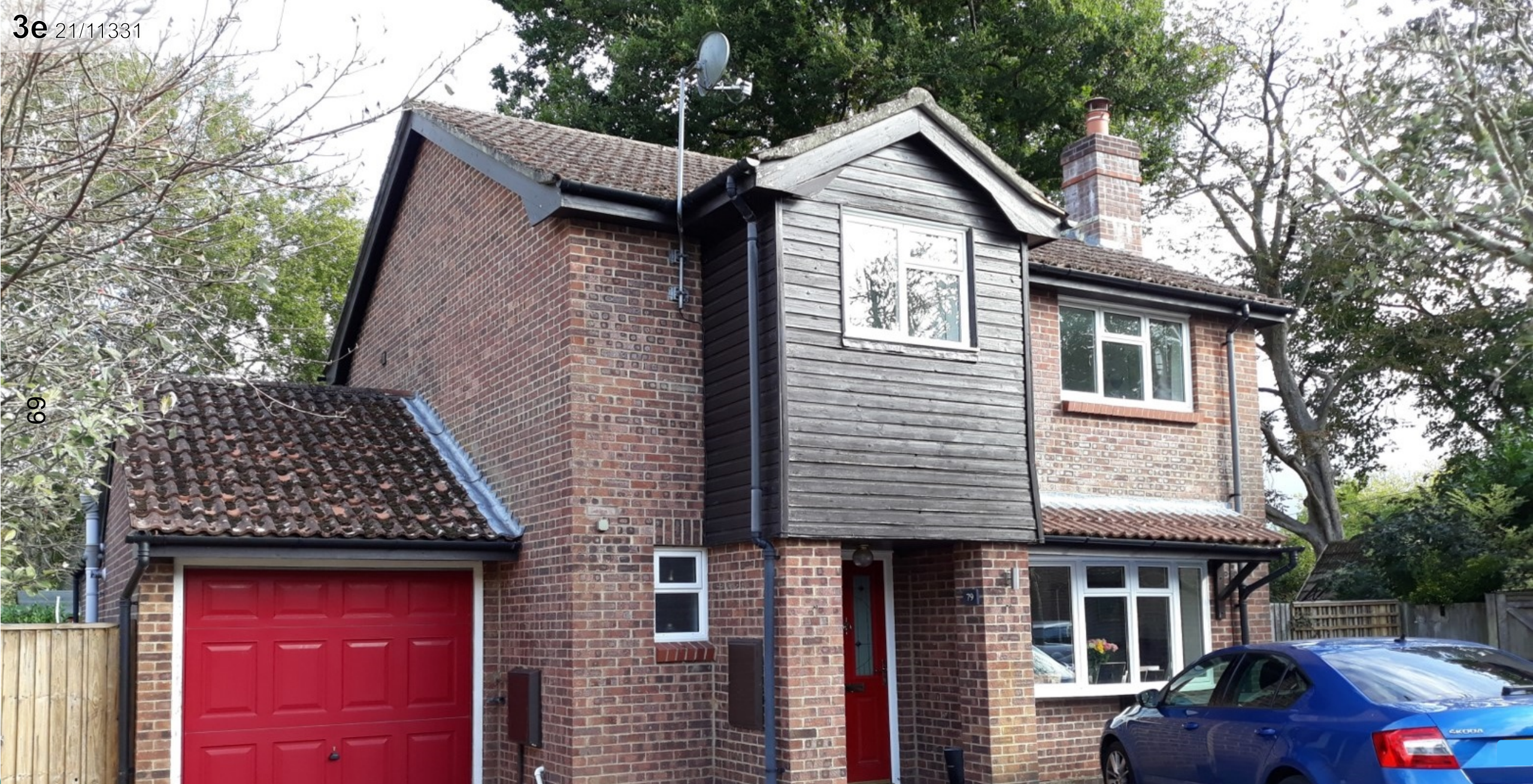
67 Front with TPO tree behind
